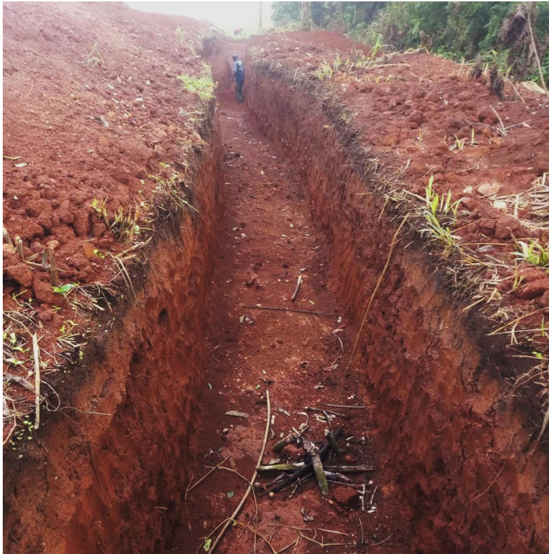
Plate 3: Trench dug in Kakooga Parish, Rwimi sub-county Bunyangabu district
