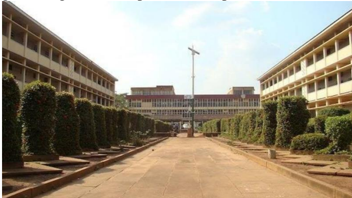
Figure 1; The Court of faculty of environment studies building, university of Nigeria Enugu campus
