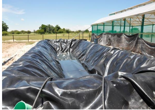
Figure 3 Dug out Ditch covered with a Dam Liner
