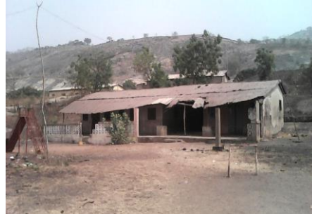
Photo 2: Partial view of the building housing the public kindergarten in the Borough of Boni Shot: Kotchoni, January 2017
